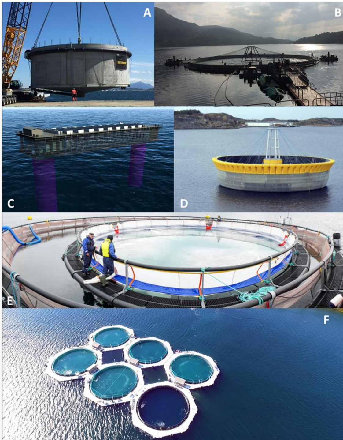
Figure 6.1-1. Different type of semi-closed systems in the sea: A) “Salmon Home #1” concrete tank (photo: Jelena Kolarevic, Nofima); B) Neptun (photo: Aquafarm Equipment); C) Preline (photo: Lerøy); D) AgriMarine (photo: Per Gunnar Kvenseth); E) FlexiBag (photo: Nekton havbruk AS); F) AquaDesign (photo: AquaDesign AS). Photo C) is reproduced with permission from Klemet Steen, Lerøy, photos D) and E) are reproduced with permission from Maria Sørøy, Smøla Klekkeri og Settefiskanlegg AS and photo F) is reproduced with permission from Anders Næss, AquaDesign AS.
